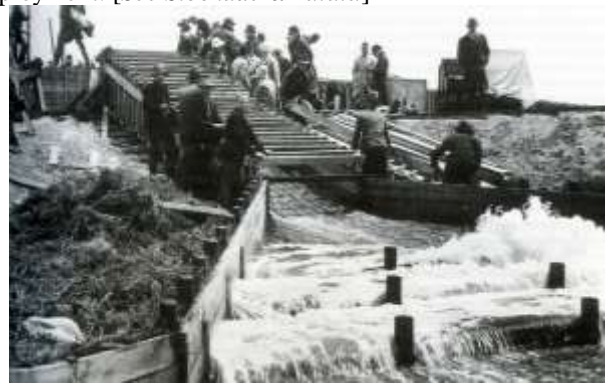
ICI works at Dry Creek - 1936
