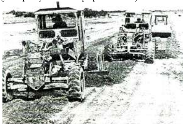
Upgrading the Dukes Highway
