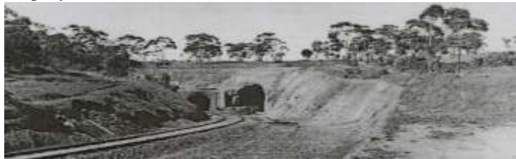
Old and New Railway Tunnels near Eden Hills - 1927
