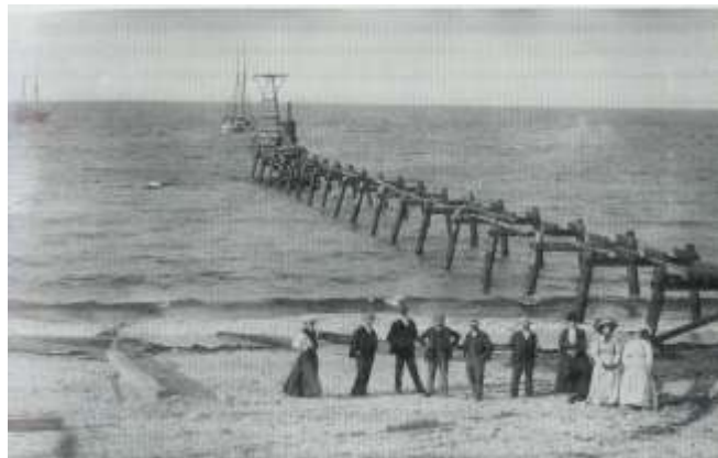
Port Neill Jetty under construction
