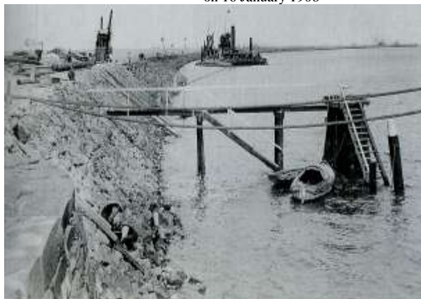
Construction underway at Outer Harbour - circa 1906
