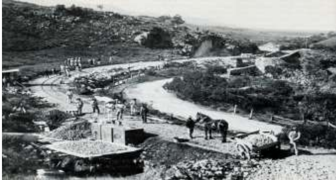
Work in progress on a cutting within Pichi Richi Pass
