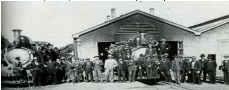
Quorn Railway Station Sheds – circa 1880
