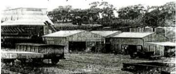
the Railway Department in spending £15,000 for the purchase of a quarry and the erection of stone crushing works which will permit ballasting being undertaken in the future at less than one half the cost entailed in the past':
