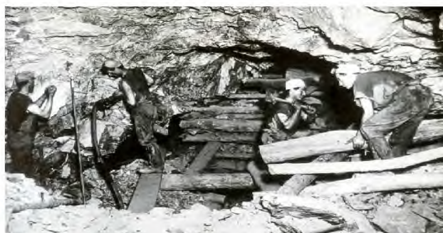
Timbering in a wide stope in the Wallaroo mines in 1916
